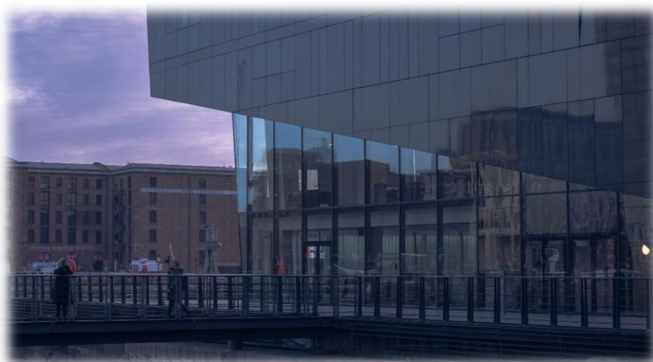
Mann Island Building, háttérben a Royal Albert Dock
